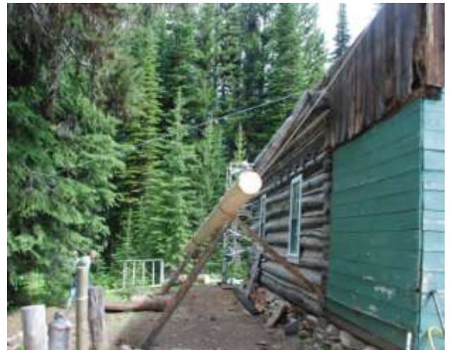
Raising the purlin
