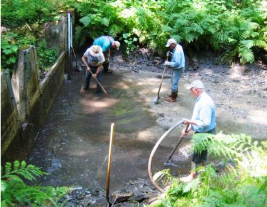
L-R: Hank Jones, Jim Burns, John MacKinnon and Carl Gidlund clean silt from the settling pond at the Benton Creek gauging station
