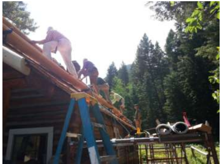
The whole crew on the roof.
