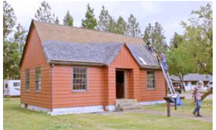
The Admin building getting the finishing touches.
