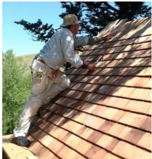
Mike on the roof, finishing up.
