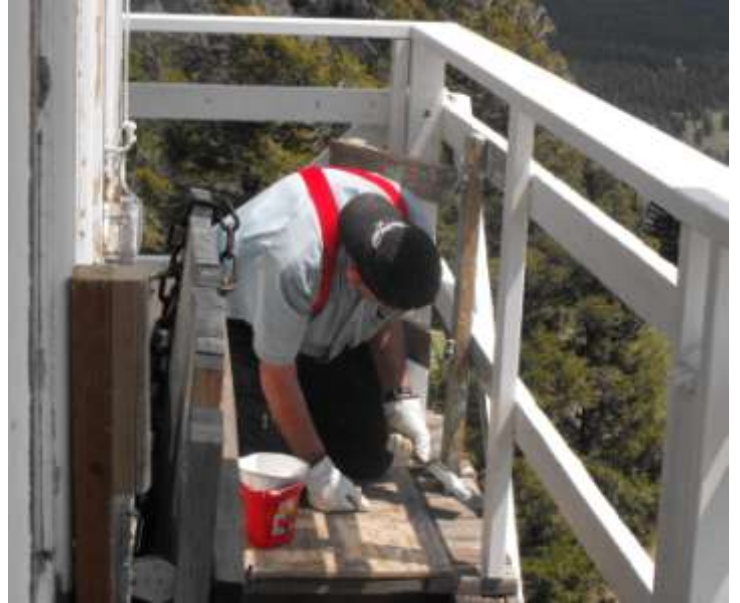
Spud working on the deck
