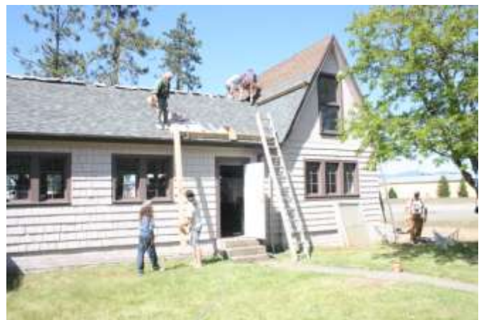
The crew working on the loft roof.
