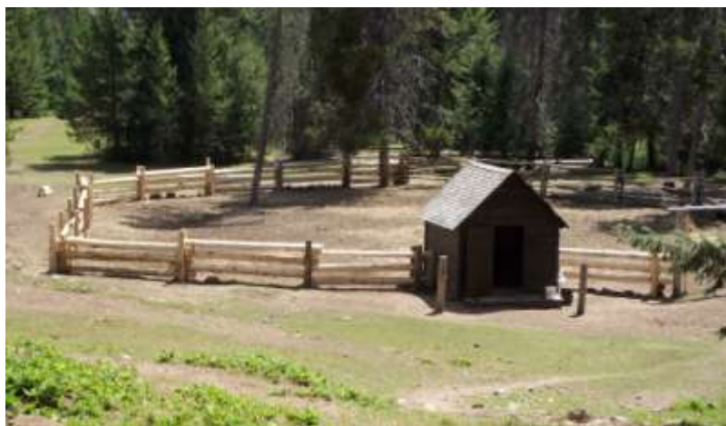
The finished corral.
