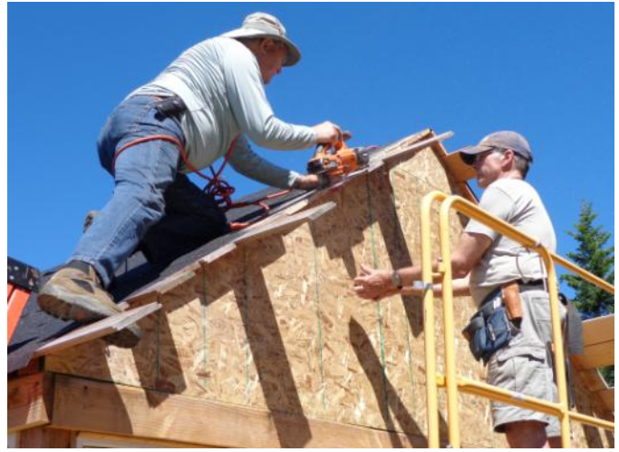
Bob Smee and Bob Denner trimming the roof.
