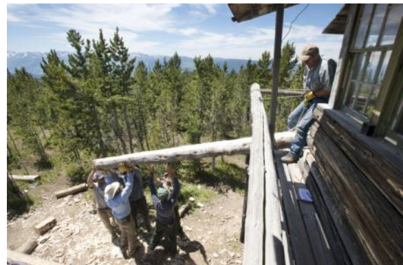
Jacking up the window sill plate: Jack Sterling, Bill Hesketh and Bob Beiermann
