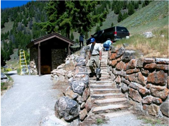
Gary and Digger doing a little masonry repair.
