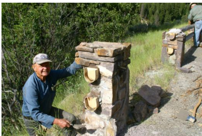
Wild Bill prepping the masonry for the rails.
