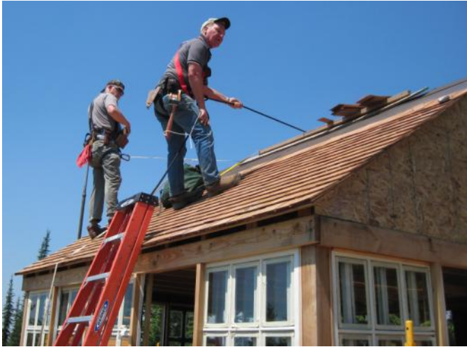
On the roof: Dave Blakely (L) and Terry Egan
