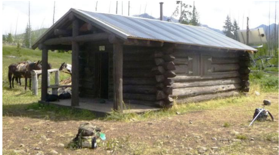
The Cache Creek Cabin with a new roof.
