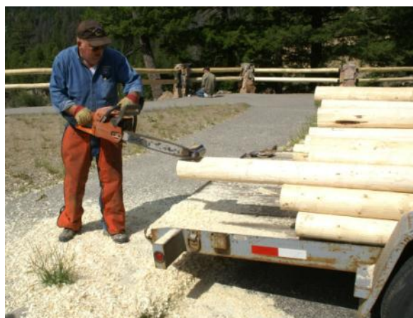
Digger using his chainsaw planner to prep the rails. Larry putting in rails in the background.
