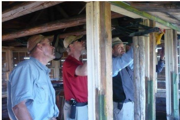
Jacking up the window sill plate: Jack Sterling, Bill Hesketh and Bob Beiermann
