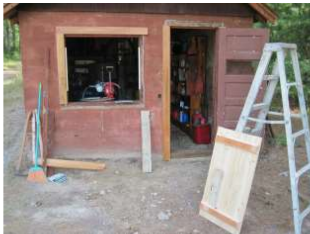
The fuel shed before work started.
