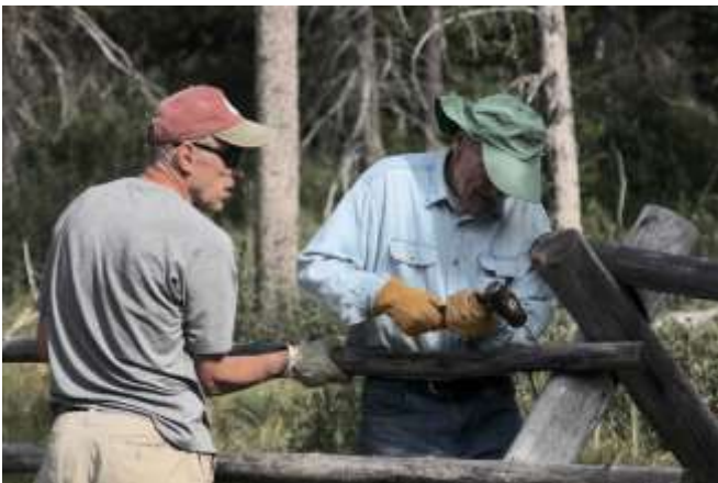
Mark and Dave working on the jack-leg fence.
