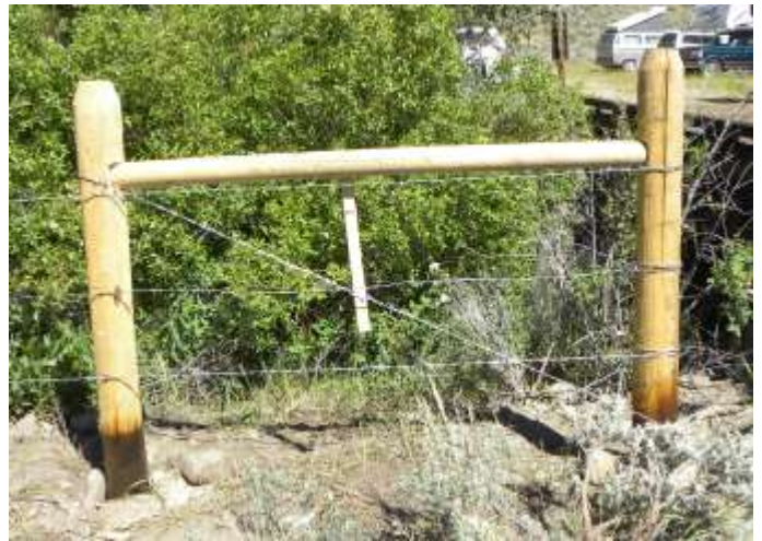
A new "H" brace ready to go.
