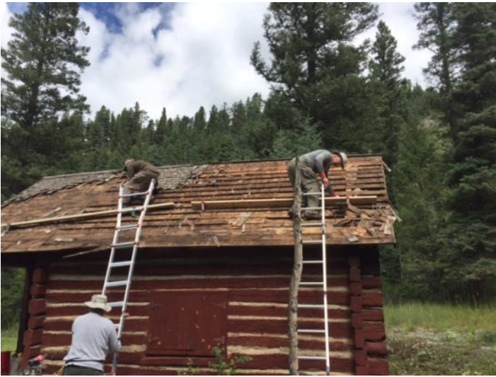
Mark and Alan removing the old roof.
