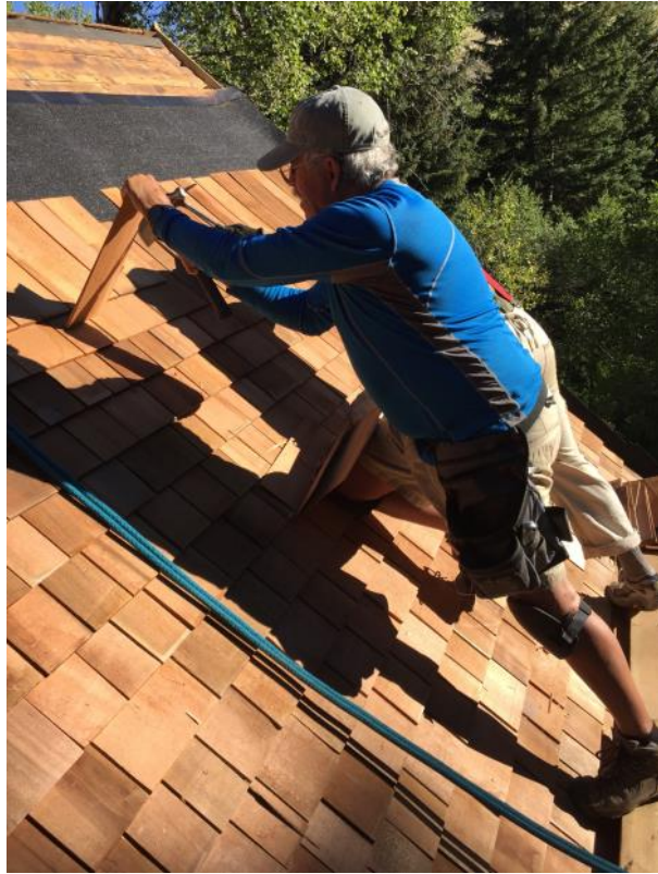
Above: Bill Hutcheson splitting a shingle to finish the row.
