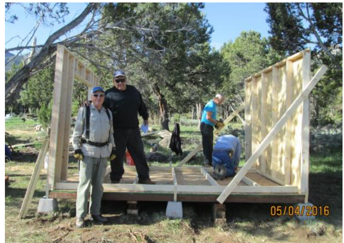
The walls are framed. L-R: Doug, Chuck, Tom Digger.
