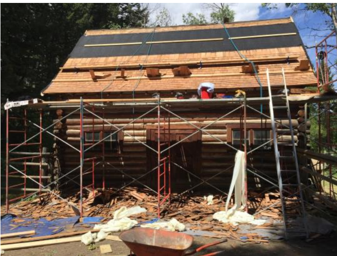
The project about half done.
