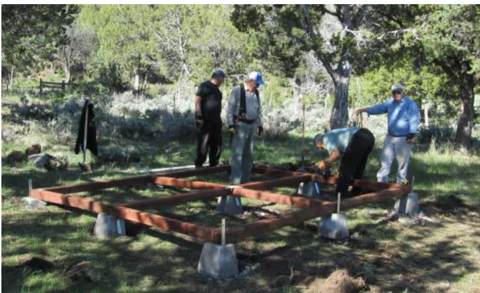
Laying the framework.
