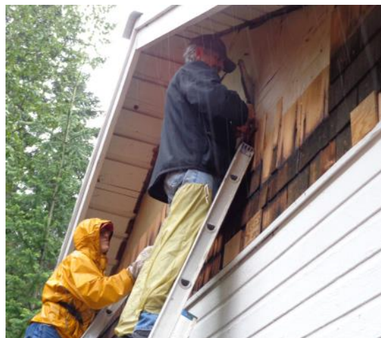
Hank and Rich removing shingles.
