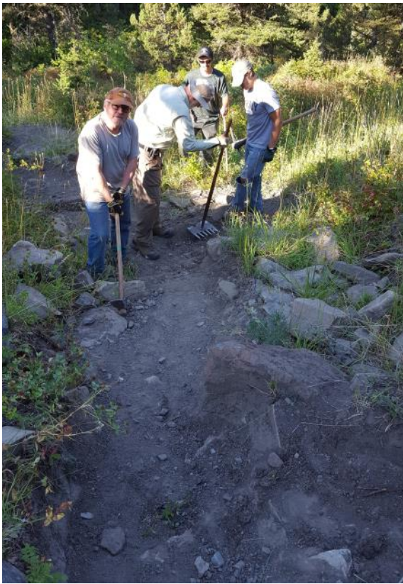
John, Lonetree, Fred working on the trail.
