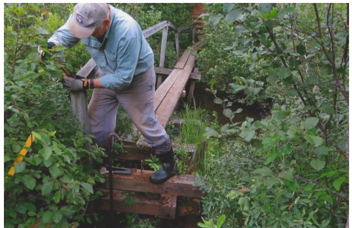
Phil Petty tearing out the old bridge.
