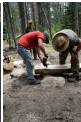
The logs were top surfaced for walking, notched for assembly, timber locked, and rock-locked in placed
