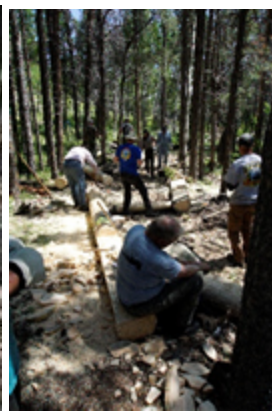
The logs were top surfaced for walking, notched for assembly, timber locked, and rock-locked in placed
