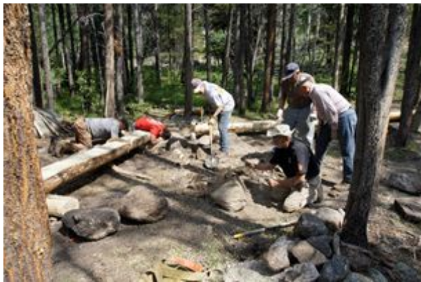
The logs were top surfaced for walking, notched for assembly, timber locked, and rock-locked in placed
