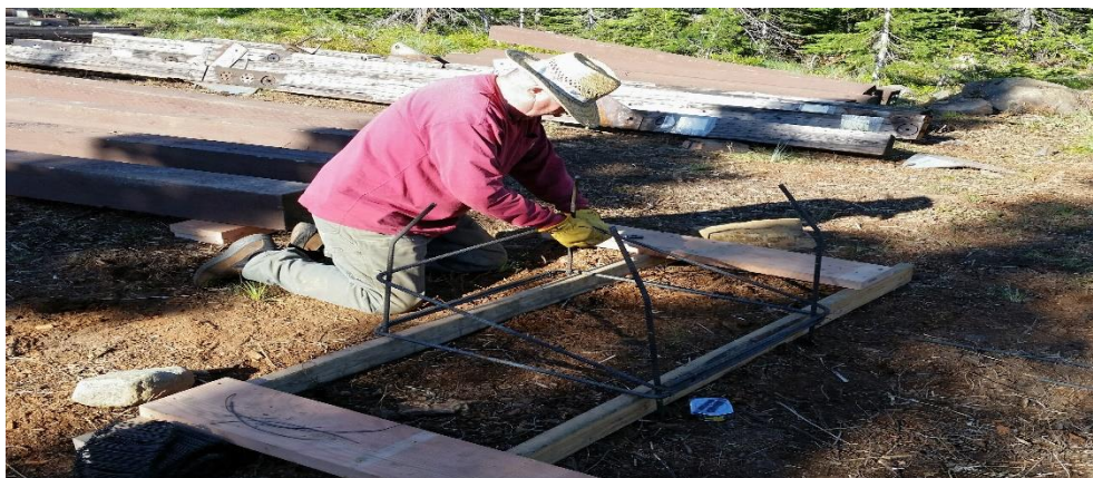
Bob Smee tying rebar.
